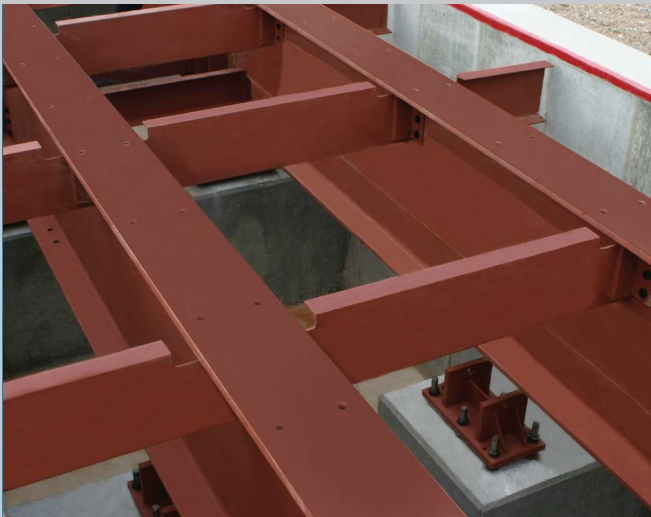
Construction of a Fairbanks A.A.R. Rail Scale involves massive reinforced concrete piers and more than 50 tons of structural steel supports to handle extreme rail car loads.
