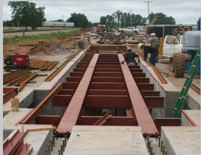
Construction of a Fairbanks A.A.R. Rail Scale involves massive reinforced concrete piers and more than 50 tons of structural steel supports to handle extreme rail car loads.
