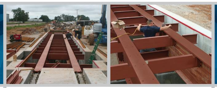
With 50 tons of structural steel and massive concrete piers, the A.A.R. Combo Scale's reinforced concrete deck with recessed rails is built to handle both rail car and truck loads.
