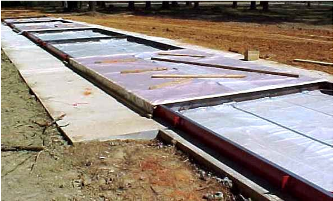
The scale assembly is ready to pour.
