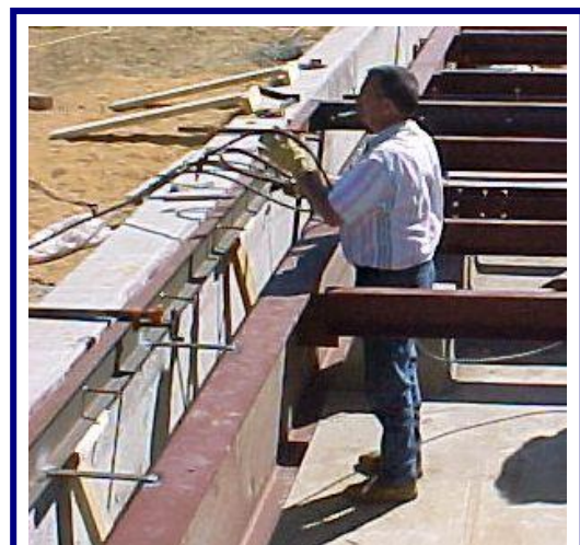
Once the bridge is completed, install the Deck Channel flush with the Pit Coping.
