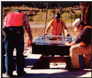
SLC scale installation
