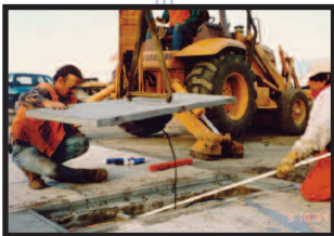
Installing the Bending Plate
