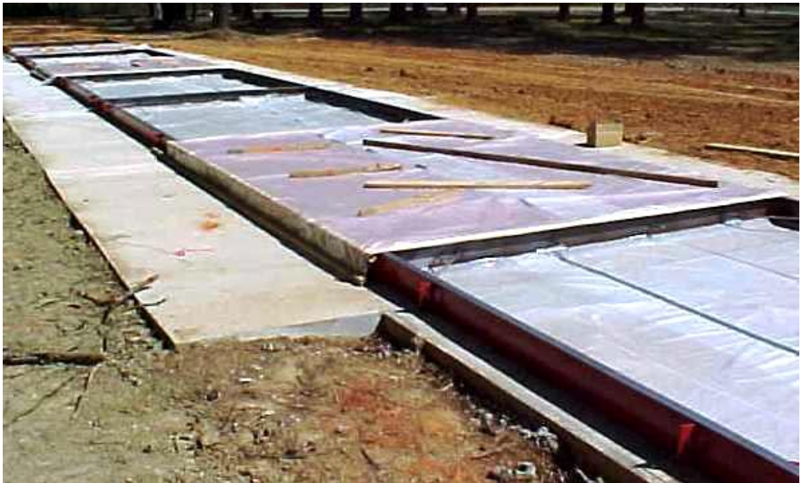
The scale assembly is ready to pour.
