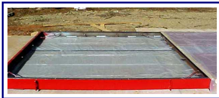
Tape edges of the concrete frame.
