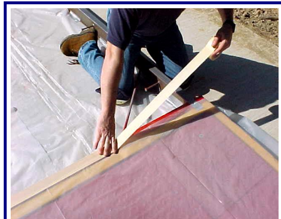
Cover decks with plastic.
