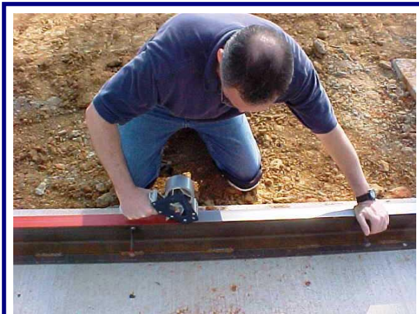
Tape edges of the concrete frame.
