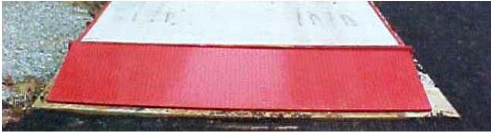
Bolt the Ramps to the Approaches
